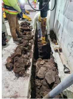
get to work. The general contractor started by saw cutting an approximately 2-foot-wide section in the 6-inch-thick (15-centimeter) floor slab running the length of each new grade beam to expose the soil below. However, plans quickly hit a snag when the crew discovered a layer of urban rubble less than a foot below the slab.
